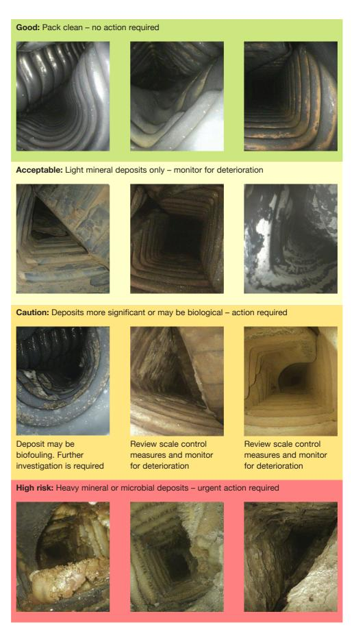
Figure 1.6 Cooling tower pack boroscope pictures
