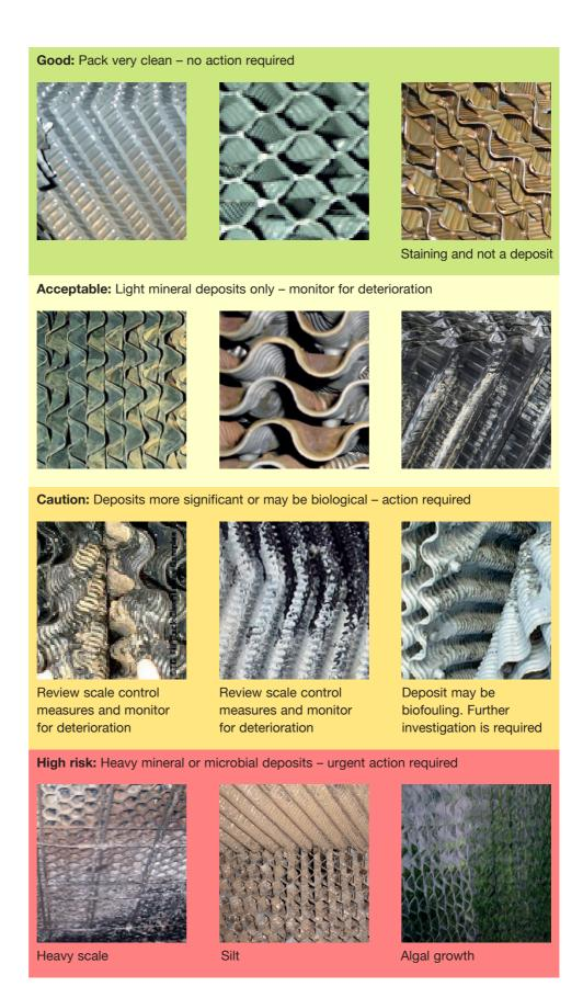
Figure 1.5 Cooling tower pack photographs
